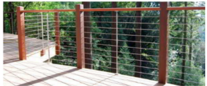
(Above) Cable railing with timber posts and handrail.
