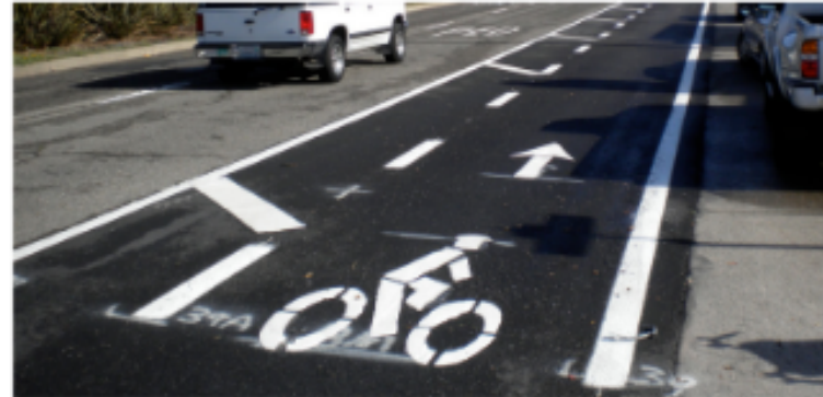
The use of pavement markings delineates space for cyclists to ride in a comfortable facility.
