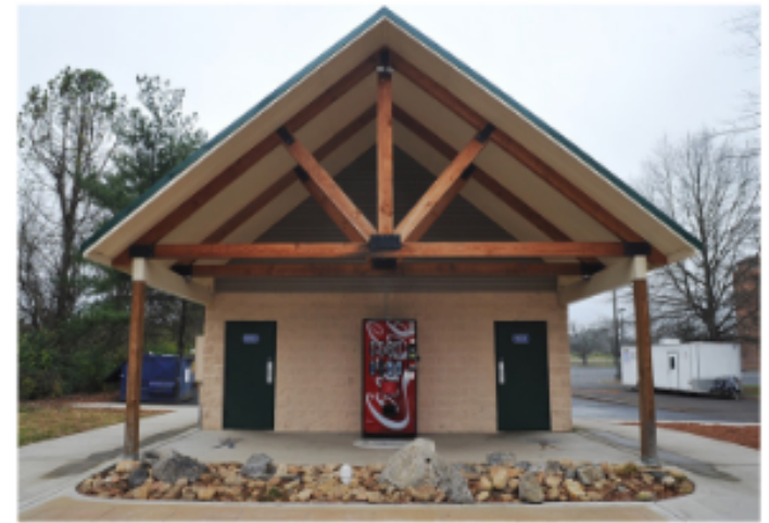
(Above) Restroom example.
