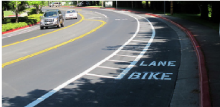
The use of pavement markings delineates space for cyclists to ride in a comfortable facility.
